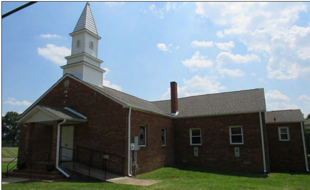
Photo 11: Zion Hill Methodist Church (GF8730), North Oblique.
