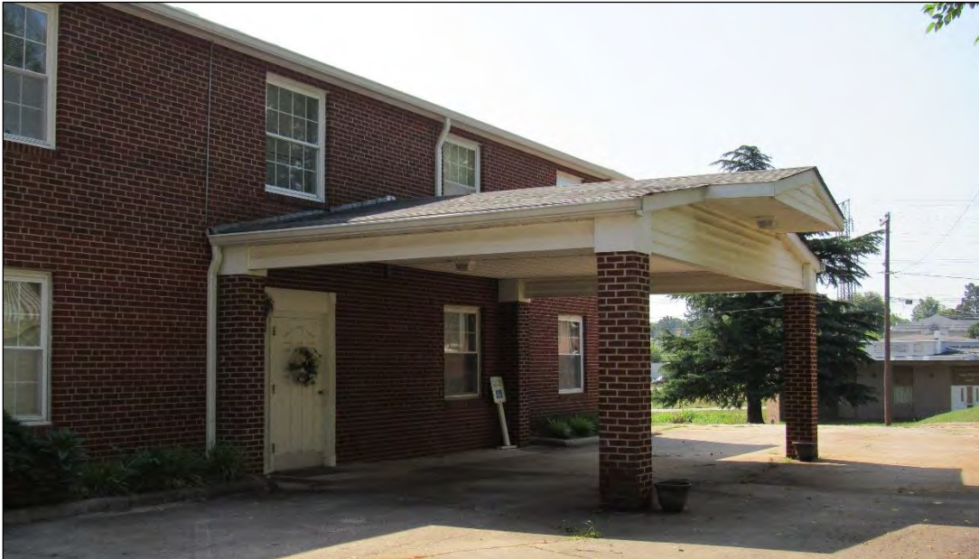
Photo 6: First Pentecostal Holiness Church of High Point, Porte-Cochère Detail.
