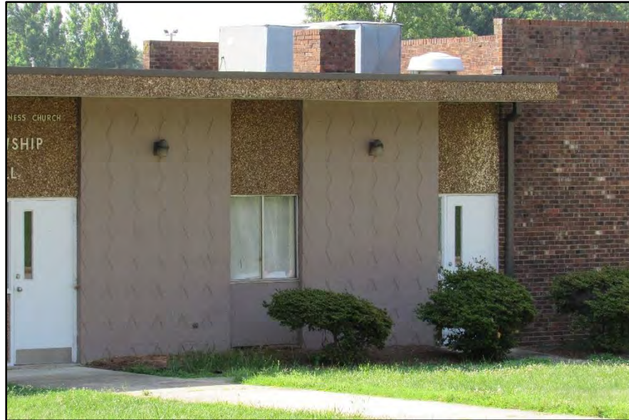
Photo 9: Fellowship Hall, Concrete Paneling on Northeast Elevation.
