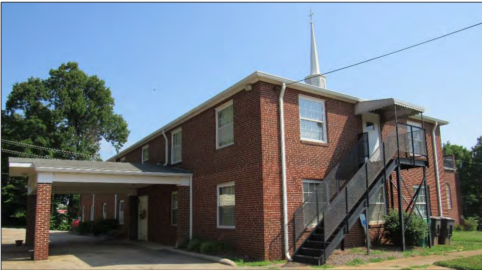
Photo 5: First Pentecostal Holiness Church of High Point, Southwest Oblique.
